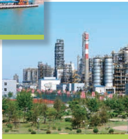
神华包头煤化工公司 Shenhua Baotou Coal-to-Chemicals branch
