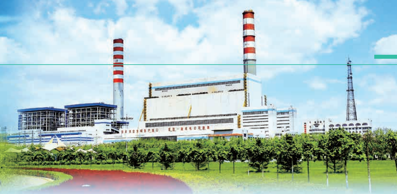
神华绥中电厂 Shenhua Suizhong power plant
